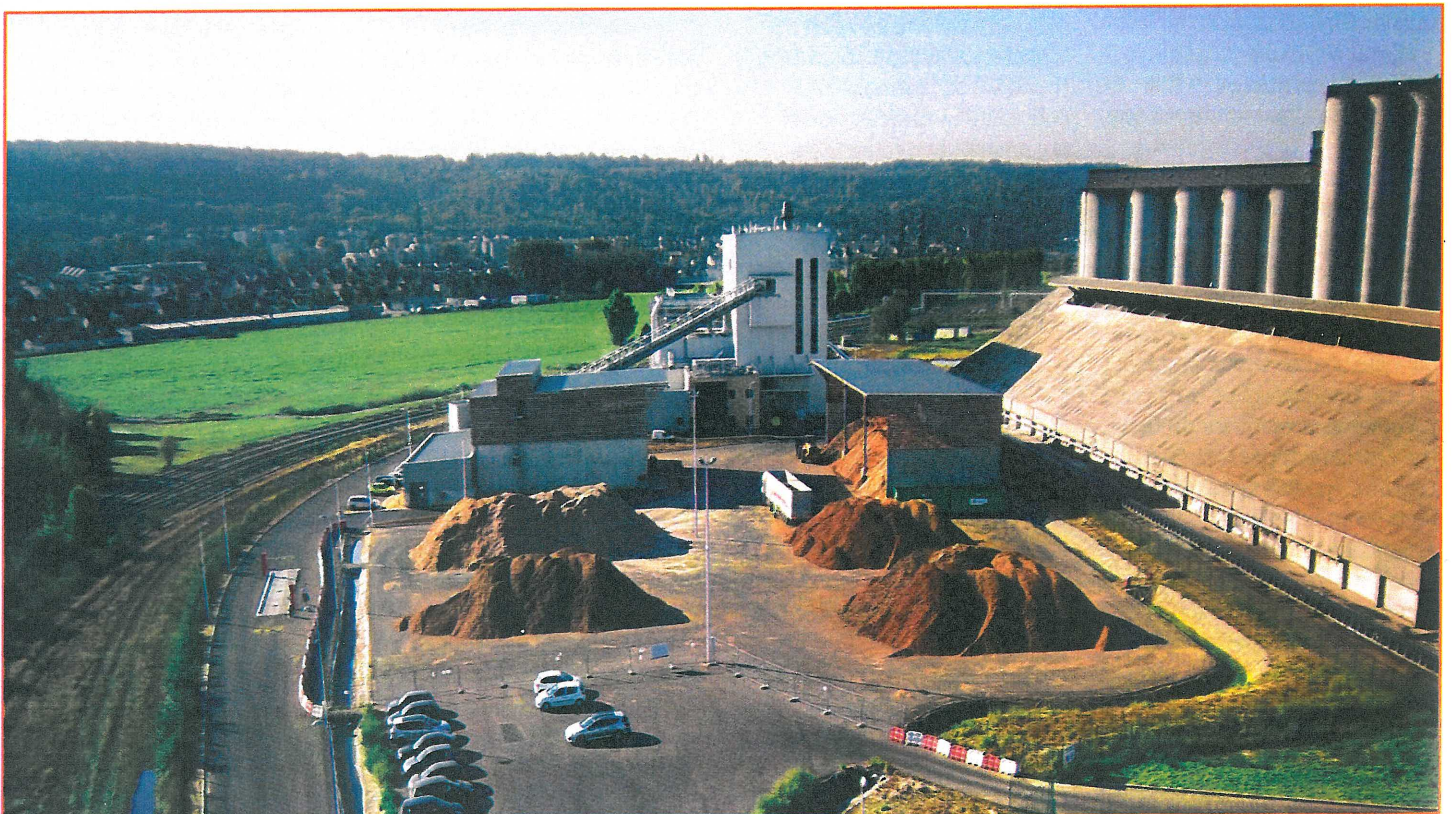
Basking in the sun: the Cofely plant produces around 64,000MWh annually
