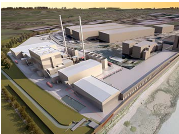
Tilbury Green Power, London, UK
